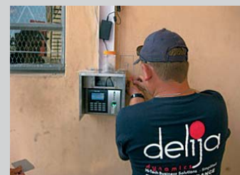
A Delija technician installing the TA100C.
